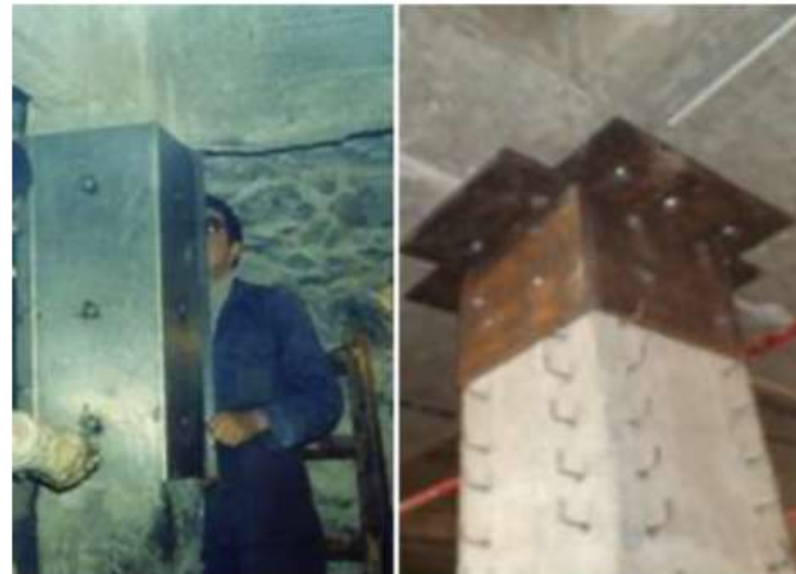
Fig. 4. Seismic upgrading with steel jacketing.
